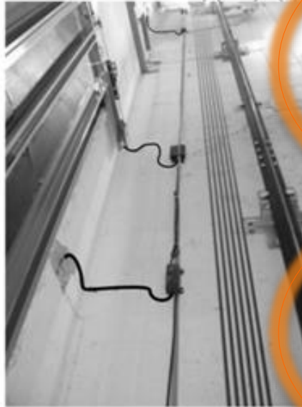
ELEVATOR SHAFT BUNDLE (CABLES AND CONNECTION BOXES WITHOUT TRUNKING)
